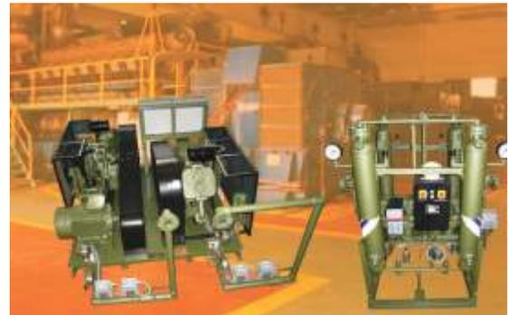
Unlike small capacity diesel generating sets which make use of batteries to start the sets, these high capacity power plants make use of high pressure starting air system to crank the engine. Compressed air at 30 bar or 40 bar is used when the diesel engine has to be started in the absence of electric supply from the power grid.
