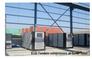
for achieving production efficiency and energy savings at its new production lines. ELGI had recommended its tandem model with the capacity of 815 cfm at 9 bar g for their newly expanded 300000 tonnes-per-annum (TPA) Rebar mill plant.
